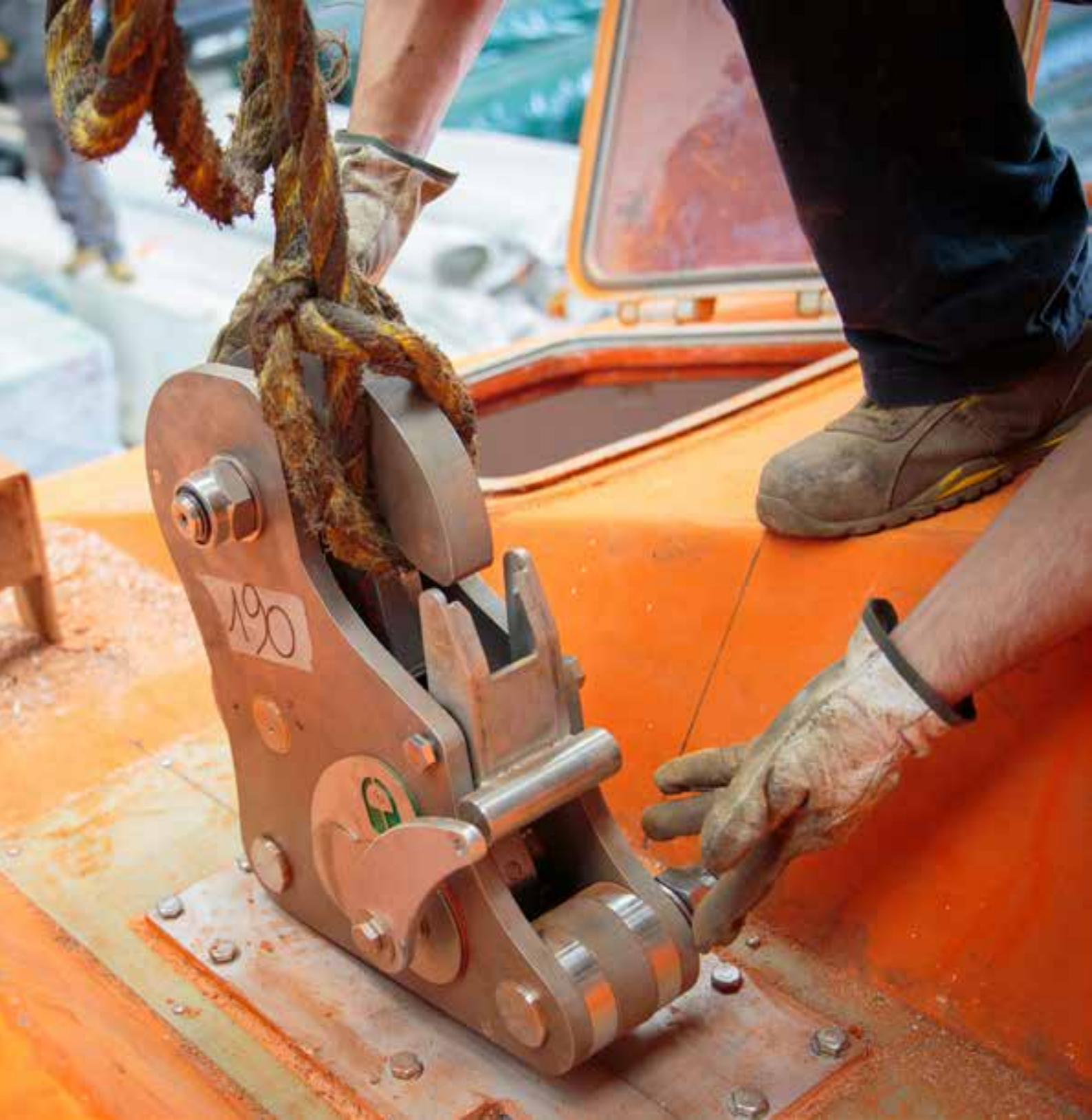
Lifeboat release and retrieval systems replacement
